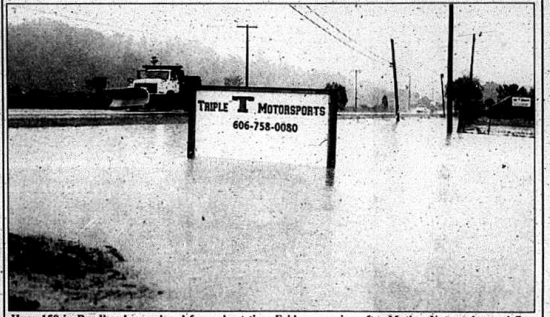
Hwy. 150 in Broadhead was closed for a short time Friday morning after Mother Nature dumped five inches of rain in the area in about an hour.
