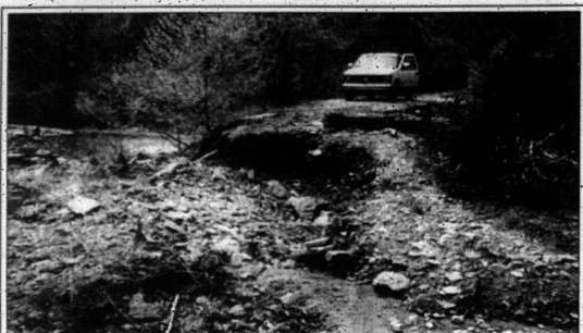
County roads have been heavily damaged by recent heavy rains. Officials with the Federal Emergency Management Agency will be in Rockcastle Thursday (today) to assess the damage.
