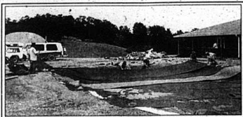
Students prepare liner for pond in front of center
