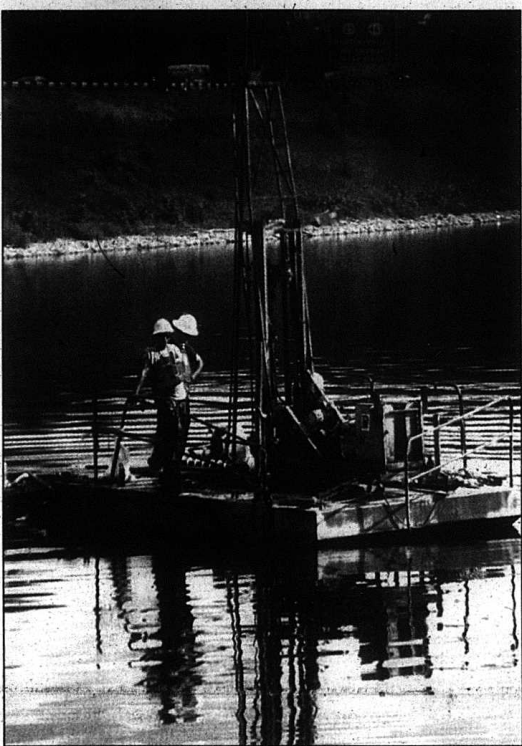
Engineers were busy on Monday core drilling around the intake valve at Lake Linville. Apparently, the valve, which has been in place since the lake was built in the 1960's has cracked and is not putting enough water into the water plant.
