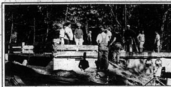
First day of cabin building
