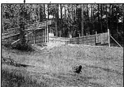
New House Under Construction
