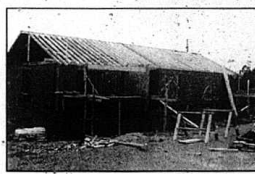
New House Under Construction
