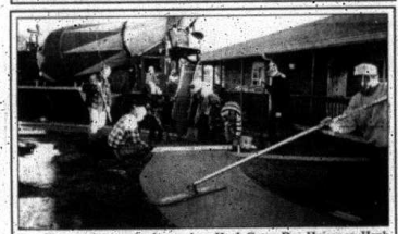
Installing a cement pond are Hank Gates, Don Huienga, Hank Loerup, Roger Ellens, Rich Brouwer and Ken Ipema.
