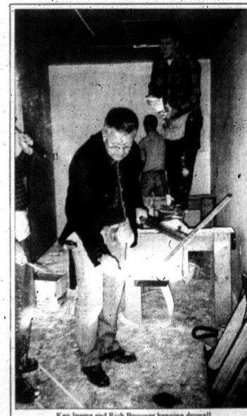
Ken Ipema and Rich Brouwer hanging drywall.
