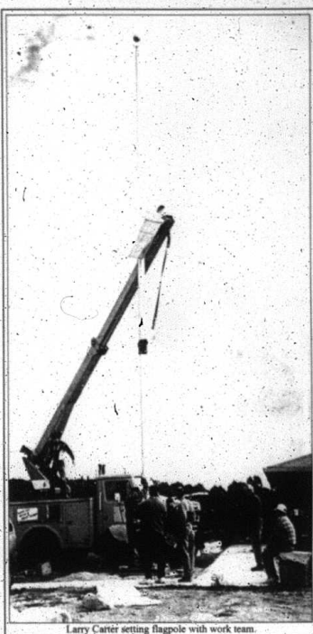
Larry Carter setting flagpole with work team.
